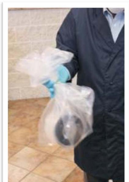
The HEPA/ULPA filter is now sealed inside of the poly liner and can be disposed of according to local governmental laws. (*Conductive poly liners are available.*)
